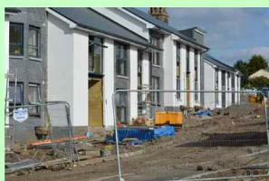
Houses nearly finished Chapel lane
