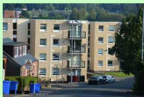
Insulation/Roughcasting New Rd
