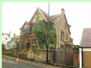
Private demolition Wallace St
