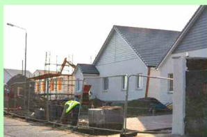
Private Development Barrmill Rd
