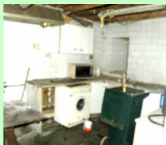
Asbestos removal Portland
